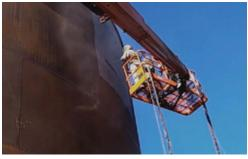
\*Production and consumption rates may vary based on nozzle size, pressure at the nozzle, standoff distance, abrasive metering, equipment quality, surface type, coating type and thickness. The blasting rates are achieved by setting the nozzle pressure to operate within the range of 95 psi – 100 psi. GMA will work with you to produce optimum performance on blasting jobs, reducing time and cost, and producing the best surface result for any coating.
